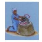
Step 7: Mark out the entrance of the stove, making it round on the top and shaping a little platform for the wood in front of the entrance. Smooth out the edges of the entrance and the surface of the stove.
